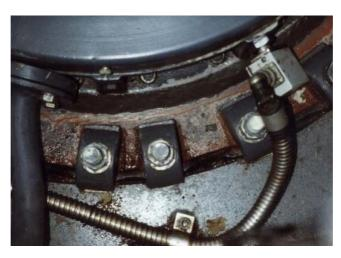
At the on-load tap changer of a large transformer oil was penetrating through cracks between the top and the on-load tap-changing equipment. The direct-MM-bonding method was used to solve this repair problem. It was carried out with MM-metal oL-steelceramic and Hardener red and afterwards Hardener yellow.
