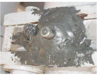
A damaged power transformer located in a steel plant has been repaired by using MM-metal oL-steelceramic and Hardener yellow.
