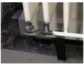
The welding at 19 places of transformers had micro cracks and blowholes, where oil exuded. First the paint has been removed with an electro drill equipped with an abrasive tool and the metal has been cleaned at the defective areas. Then MM-metal oL-steelceramic with Hardener red and afterwards Hardener yellow was applied. After checking the tightness of the repaired areas the corresponding areas have been painted over again.
