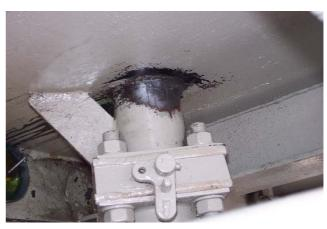
Oil exuded through micro cracks caused by vibration in a defective welded seam. The leak of oil has amplified after unsuccessful attempt to execute repair by usual welding. Then it was decided to carry out a repair by using the "direct-MM-bonding"- technology with the help of MM-metal oL-steelceramic and hardener red followed by a second layer of MM-metal oL-steelceramic with hardener yellow.
