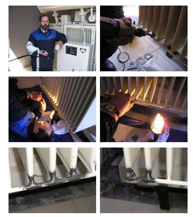
The welding at 19 places of transformers had micro cracks and blowholes, where oil exuded. First the paint has been removed with an electro drill equipped with an abrasive tool and the metal has been cleaned at the defective areas. Then MM-metal oL-steelceramic with Hardener red and afterwards Hardener yellow was applied. After checking the tightness of the repaired areas the corresponding areas have been painted over again.
