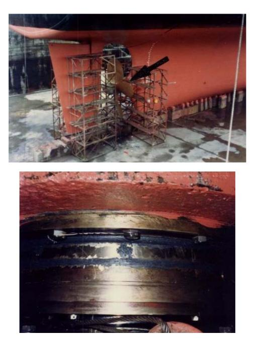
Repair of a leaking simplex compact packing. The repair was difficult due to oil pouring out of the repair site. Therefore it was decided to use the direct-MM-bonding method by applying the PolymerMetal directly on the greasy surface. Here MM-metal oL-steelceramic with Hardener red was chosen.
