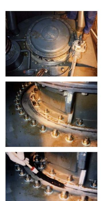
Sealing of an oil leak between the cover and diverter switch of a transformer with MM-Elastomer 95. First the oil in the transformer was drained and the surface thoroughly cleaned with MM-Degreaser Z. Finally MM-Elastomer 95 was applied using a brush.
