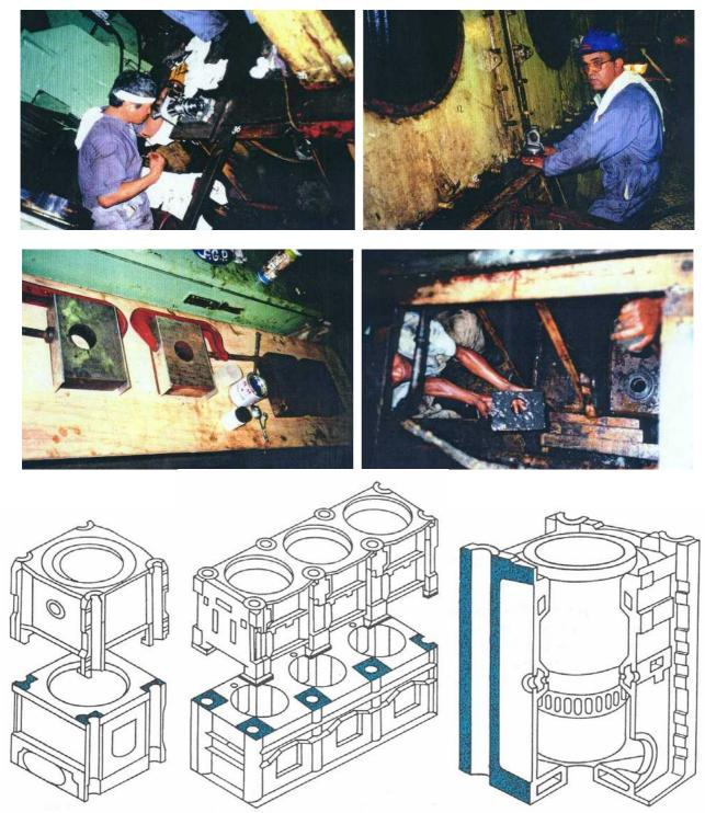
Repairing of cylinder blocks and working faces of a big marine diesel engines with MM-metal SS-steelceramic. The repair was necessary due to damages caused by big abrasion between cylinder block and working face particularly in the region of the scaving air receiver. For this type of repair the engine manufacturer recommends to use exclusively MM-metal SS-steelceramic with Hardener green.
