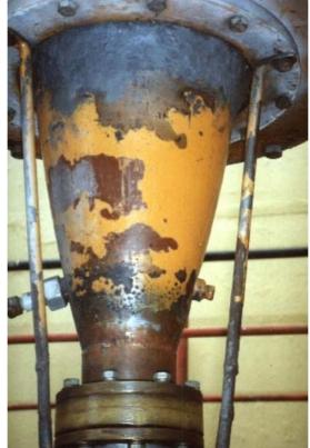
Oil flew trough a crack at the cable terminal funnel of a block transformer. The repair was carried out by the method of direct-MM-bonding with MM-metal oL-steelceramic, Hardener red and Hardener yellow.
