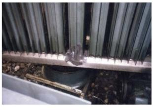
Sealing of a large transformer in a power station. The leakage was sealed with MM-metal oL-steelceramic and Hardener red using the direct-MM-bonding method. Then a layer of MM-metal oL-steelceramic and Hardener yellow was applied to the first layer.
