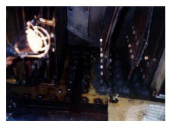
The surface of a transformer between copper plates and fibreglass coating showed several oil leakages. The repair has been affected using the direct-MM-bonding method with MM-metal oL-steelceramic combined with Hardener red and Hardener yellow afterwards.
