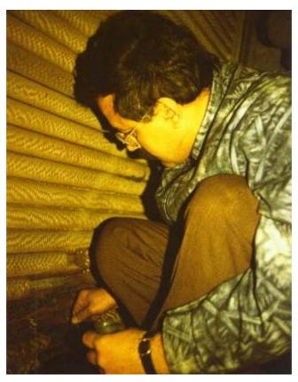
Sealing of a cooling water pipe made of steel without switching off the plant. Cause of the damage was material fatigue. The repair was carried out with MM-metal UW with Hardener UW3 and MM-Fabric tape (glass fibre).
