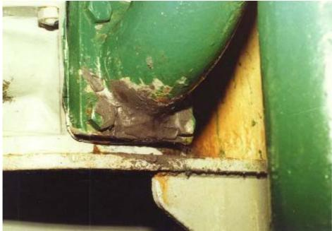
Repair of a water piping which was under pressure by using MM-metal UW and Hardener UW3. The sealing has been carried out while water was still escaping.
