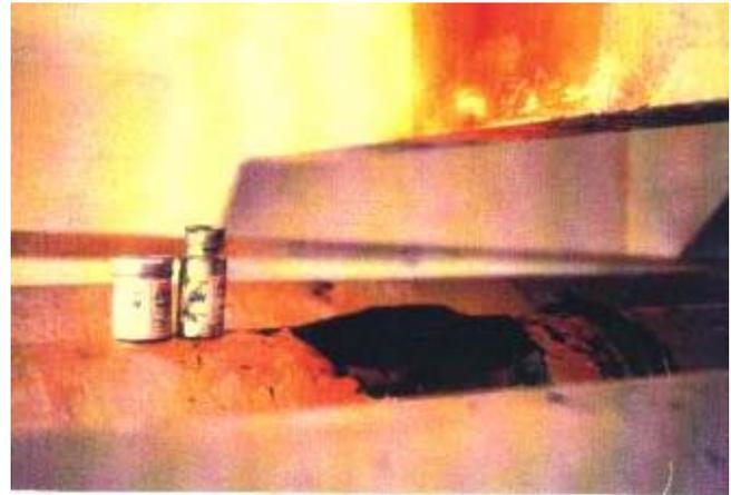
A leakage in a cooling pipe was sealed without reducing the water pressure. The repair was carried out with MM-metal UW and Hardener UW9.
