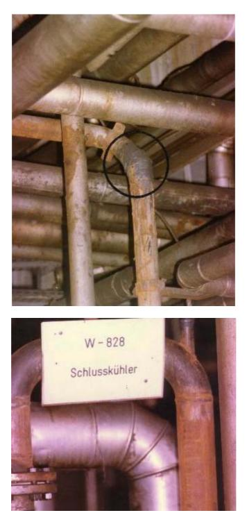
Sealing of a cooling water pipe in the high-hazard area of a high-pressure water installation without interrupting operation. The leakage was a 5 cm long crack at a water pressure of 2,5 bar. The sealing was carried out with MM-metal UW and Hardener UW3 without pressure reduction. Materials used were a pre-shaped metal sheeting and MM-Fabric tape (glass fibre).
