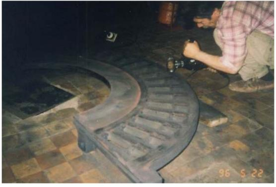
Reconstruction of the sealing surface of the cover at a turbine. The repair was carried out with Ceramium, liquid and Hardener CE at an electric generating station.
