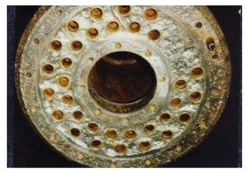
Repair of the soot blower compressor at a heat station by coating the additional cooler with Ceramium. The coating was affected in two steps: a first application of Ceramium pasty type, afterwards a second application with Ceramium liquid type.
