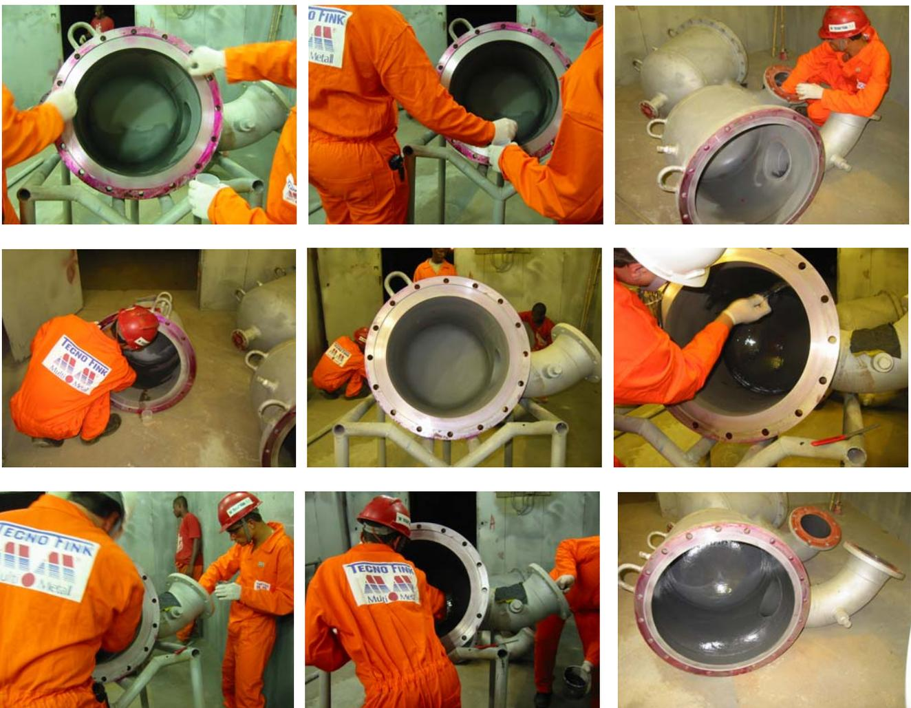
Several defective covers of a heat exchange system were repaired with VP 10-017.
