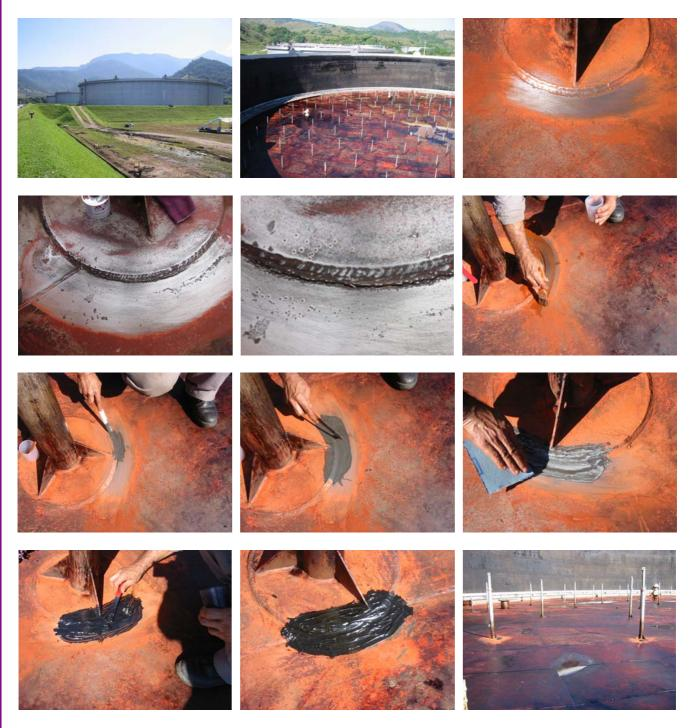
Several holes and damaged spots respectively in the roof of a big tank at an oil refinery were first grinded and cleaned to prepare the surface and then coated with Ceramium. Then the Ceramium was grinded to rough up the surface. Finally a layer of MM-Elastomer was applied to compensate any bigger tensions.
