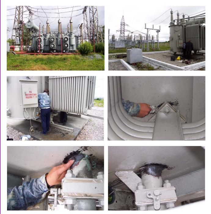
Oil exuded through micro cracks caused by vibration in a defective welded seam. The leak of oil has amplified after unsuccessful attempt to execute repair by usual welding. Then it was decided to carry out a repair by using the "direct-MM-bonding"- technology with the help of MM-metal oL-steelceramic and hardener red followed by a second layer of MM-metal oL-steelceramic with hardener yellow.
