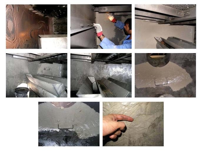
A refinery's gas washer for cleaning sour natural gas suffered from hard exposures and had massive corrosion damages in several areas. There appear high temperatures (140 °C), pressure (3 bar) and a line of chemicals (Amines MDEA, H2S, CO2, O2, various acids, ...). With MultiMetall's coating material Ceramium<sup>®</sup> CH / Hardener CH1 excellent results were achieved. Further details can be found here
