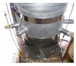
A piping made of carbon steel in a refinery had a severe leakage with benzol streaming out with high pressure (10 bar). With the help of an auxiliary construction, MM-metal oL-steelceramic and MM-metal SS-steel the leak was sealed. Here besides the common application method (trowelling) also the injection method was used.
