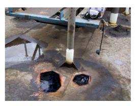
Alternatively to extensive conventional repair procedures (e.g. welding works) at floating roof tanks an expensive drain of the liquid stored in the tank can if applicable be abstained from by using a repair method with PolymerMetall<sup>®</sup>. MM-metal oL-steelceramic can be applied on problematic surfaces (contamination due to oil, fuel et cetera). The additional purpose of the flexible material MM-Elastomer is effective against tensions.
